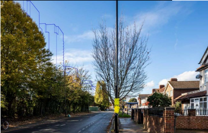
Verified View (from TVA) from east side of Park Avenue towards Blocks A1-A3 – blue stringline (black stringline behind shows new development on Merrick Road):
