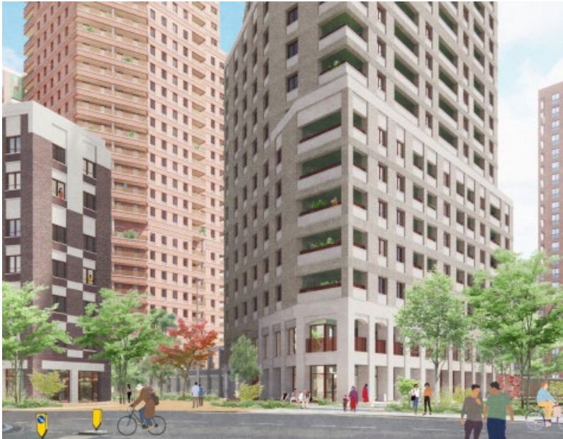
View from Merrick Road bridge towards rear of Blocks A1 – A3:
